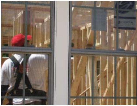
Simonton Windows being installed
