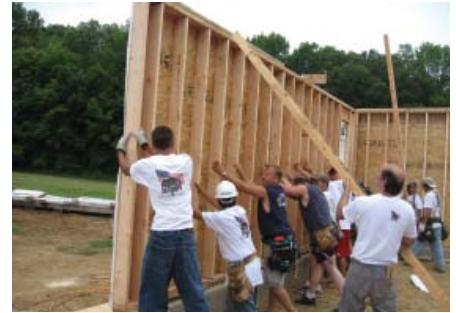
Walls going up!
