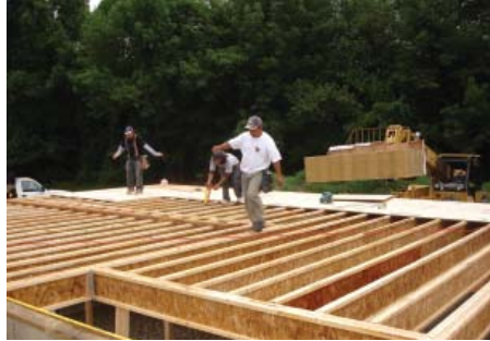
Friday morning - deck going on
